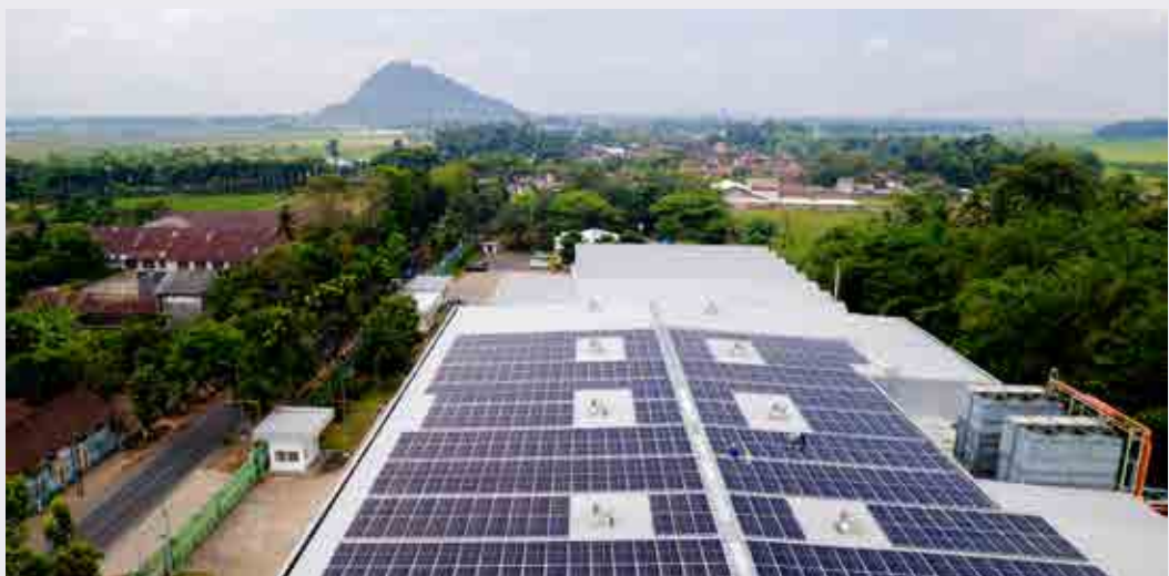
Solar panels installed on the roof of GMIT factory in Jember, East Java.
