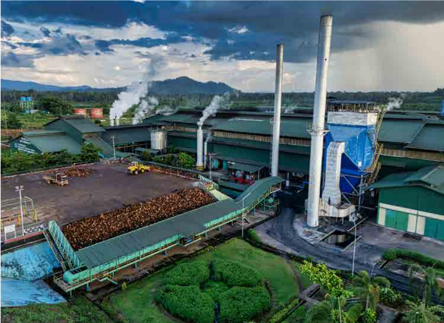
Our Palm Oil Mill at KAL, Ketapang, West Kalimantan
