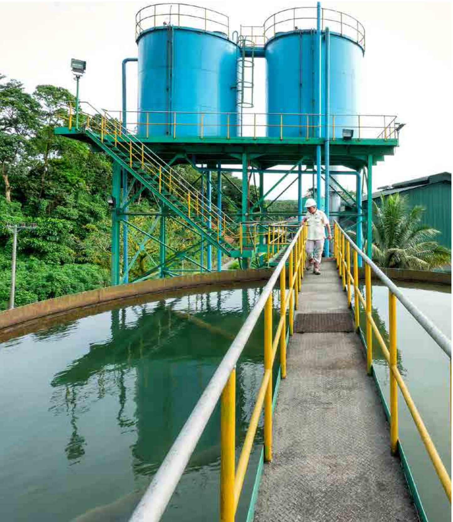
A Staff monitors water flow in the water tank at our palm oil mill.
